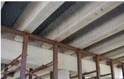
I-565 bridge girder, ready for repair
