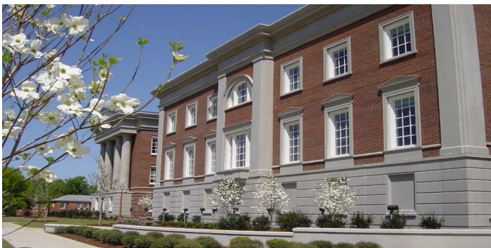
Completed, UTCA offices on second floor
