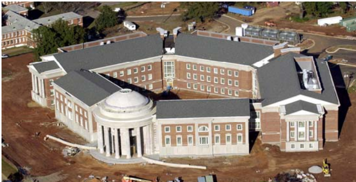
Shelby Hall under construction
