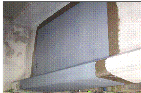
Girder after VARTM repair
