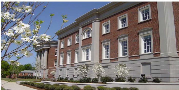
Completed, UTCA offices on second floor
